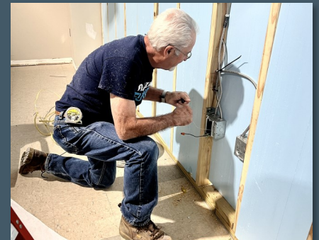
Work at the second job site
