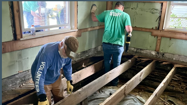
Removing old flooring
