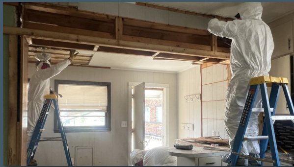
Clearing out the kitchen area
