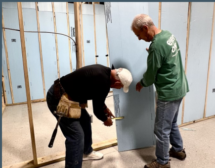
Work at the second job site
