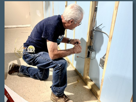
Work at the second job site
